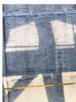
▲塗料半乾き状態
